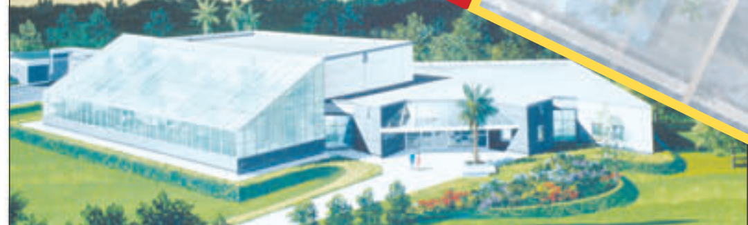
The $6.5 million laboratory is set to open this summer. The USDA's Agricultural Research Service will operate the 20,000-square-foot building.
